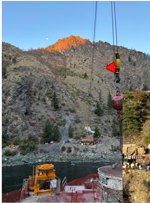
Off loading, flying, and pumping concrete for Abutment 1
