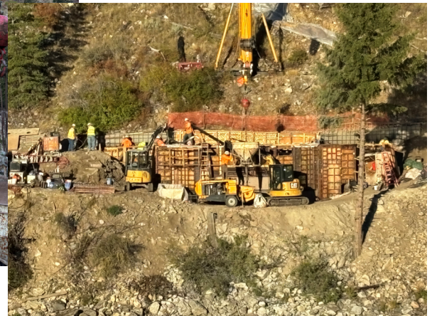
Off loading, flying, and pumping concrete for Abutment 1
