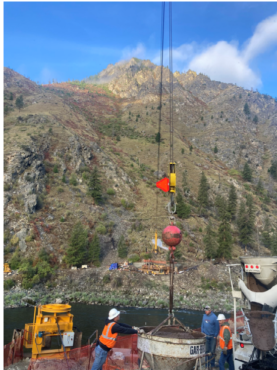
Off loading and flying concrete for Abutment 1
