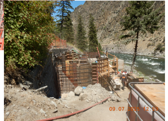
Setting forms and reinforcing steel at Abutment 1
