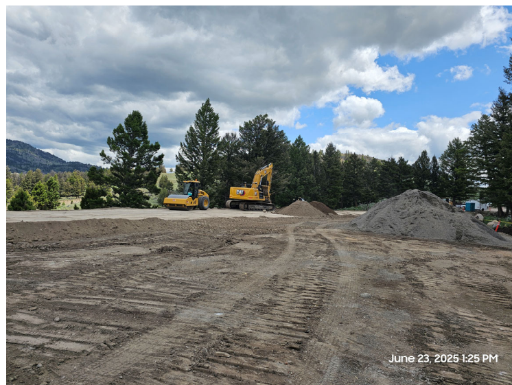
Embankment process at Abutment 2.
