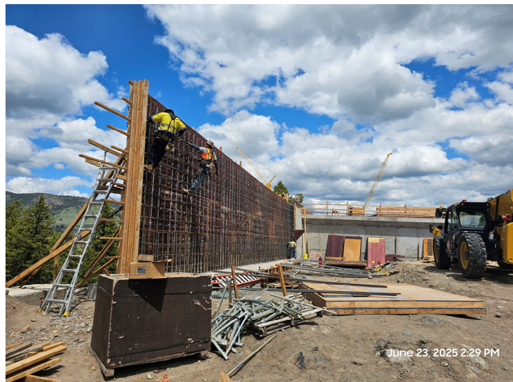
Rebar tying process for Wingwall A at abutment 1.
