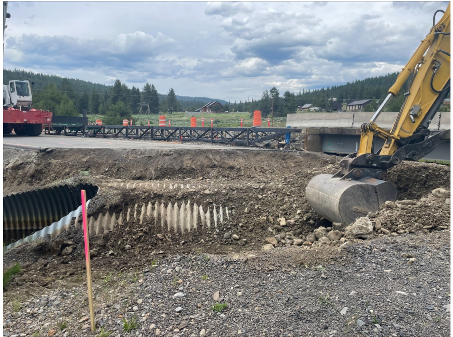
Excavation of Culvert at Bull Run #4
