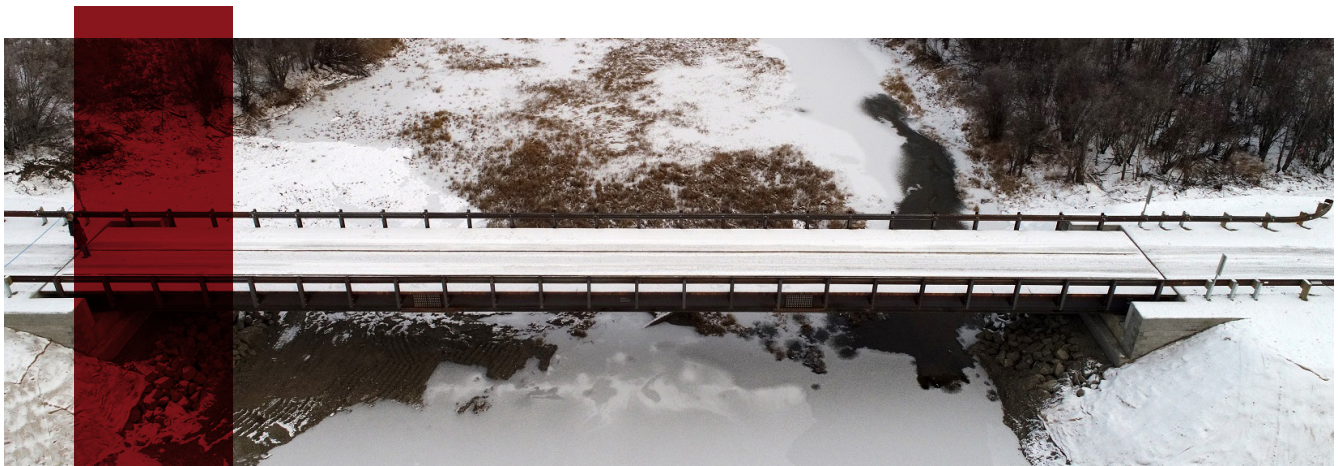
Fort Yukon Ivar’s Bridge Replacement completed. Fort Yukon, Alaska.
