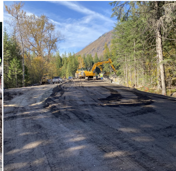
Roadway realignment work
