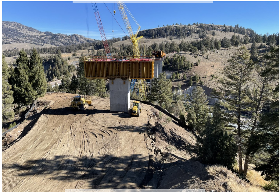
Embankment and Crane Pad at Pier 1
