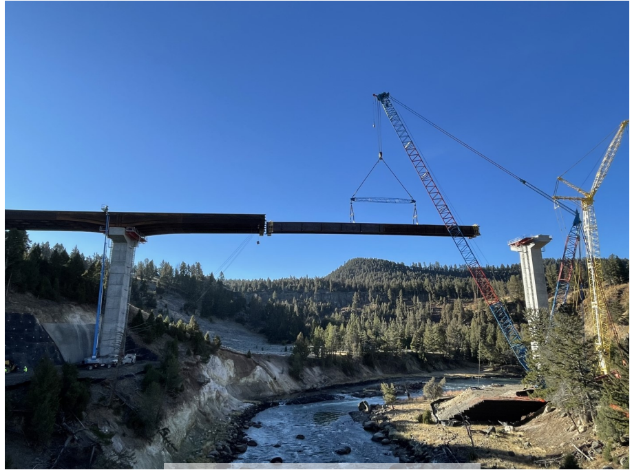
Girders Being Placed at Pier 2
