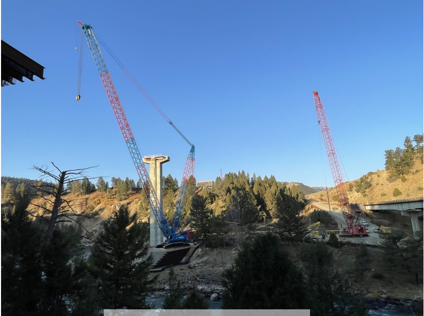
New Crane at Pier 2
