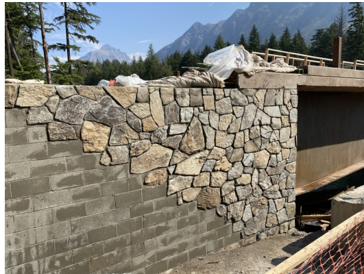
Abutment 2 masonry veneer
