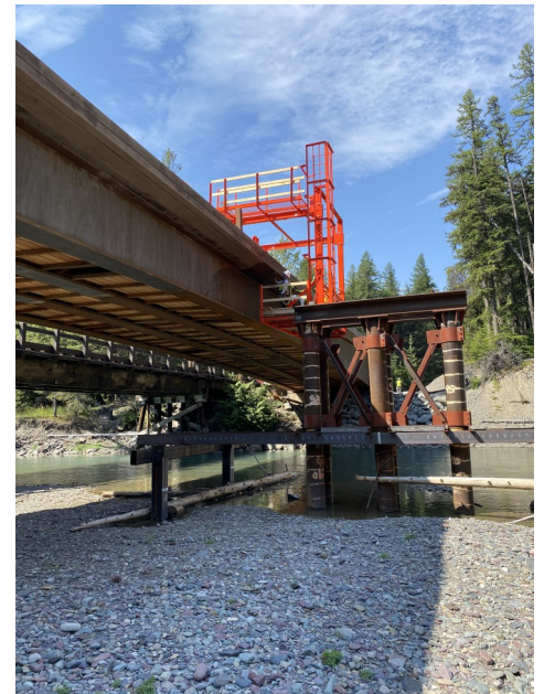
Finishing concrete overhangs
