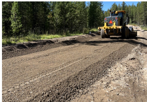
Grader Spreading the Base
