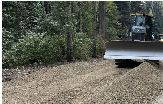
Loader Working the Surface Material
