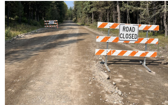
Barriers at Edge of Work Zone
