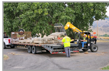
Removal of Replaced Guardrail Posts
