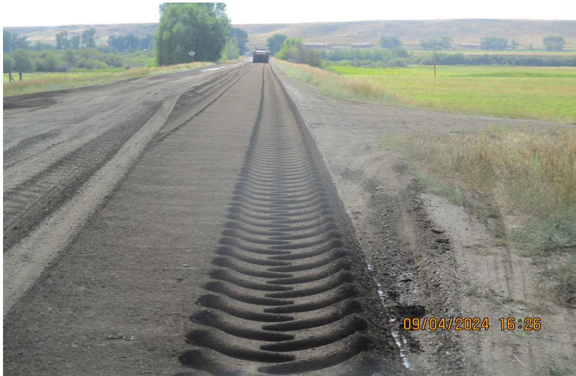
Reclaimer pulverizing roadway near MP 3.
