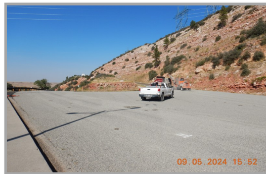
Sweeping Operations after Chip Sealing NPS 313/Upper Wappa Switchyard Road
