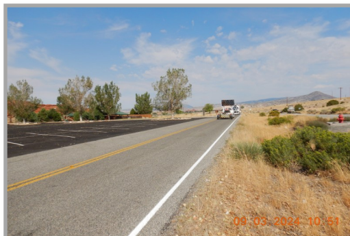
Permanent Pavement Markings on Horseshoe Bend Road
