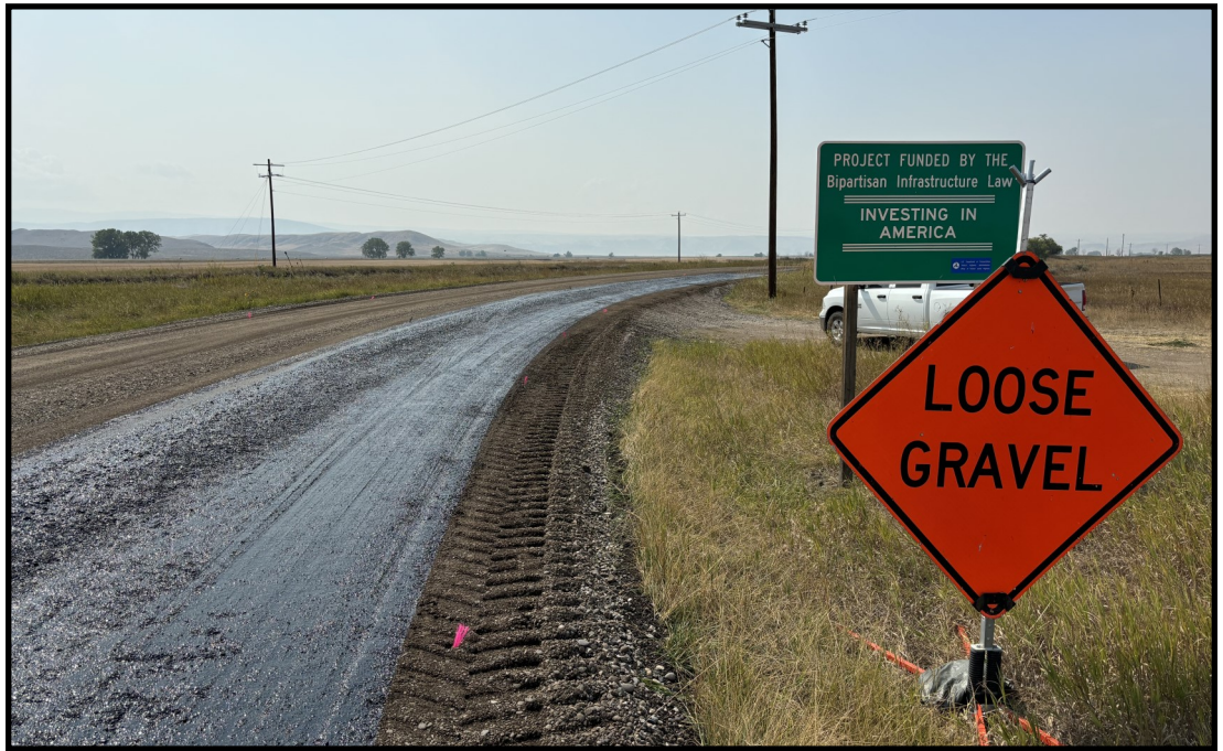
Above, a fresh layer of primer is applied to the road surface to create an optimal foundation for the upcoming asphalt application. This primer ensures better adhesion of the asphalt, contributing to a smoother and more durable finished road.
