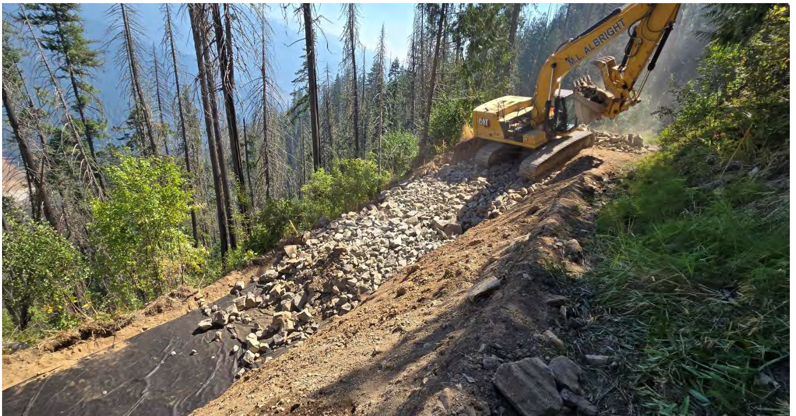
Special Rock Embankment placement, M.P. 2.52 FSR 470
