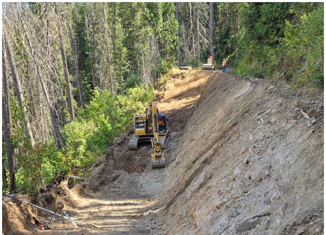
Structural Excavation for RSS M.P. 2.52 FSR 470
