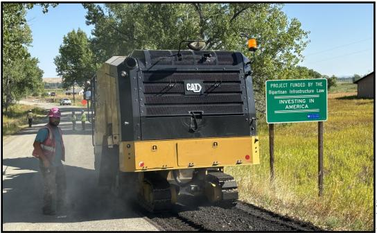
The contractor has undertaken an additional 700 feet of asphalt milling and paving preparation work as part of the project. With the addition of the remaining section of roadway, the entire length of the Warman Loop Road will be fully reconstructed.
