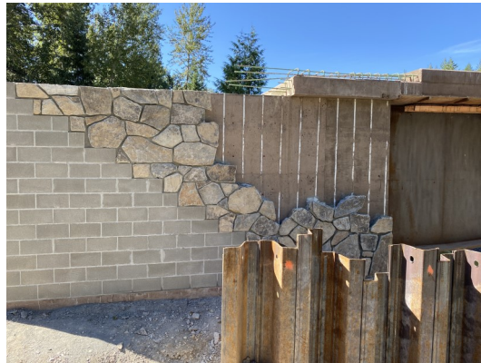
Abutment 1 masonry veneer
