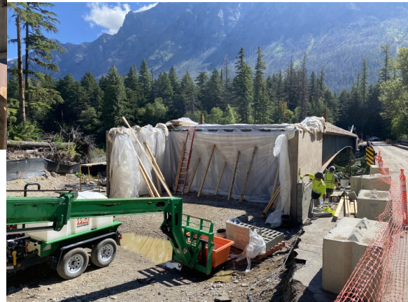
Abutment 2 walls curing
