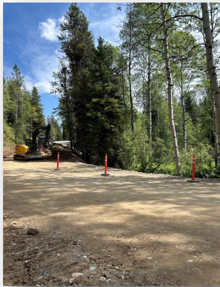
Subgrade Operations on North Fork Road
