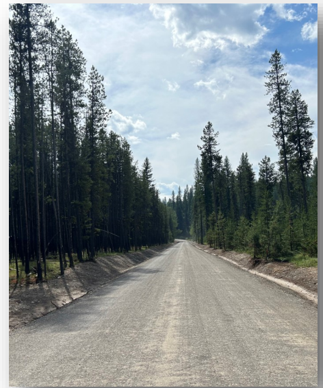
Surface Aggregate Placement on North Fork
