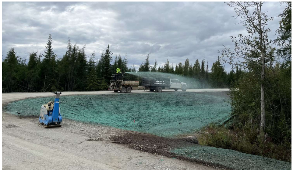
Bottom: Hydroseeding slopes.
