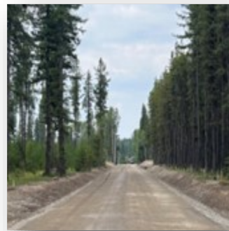
Bottom Photo: Surface Aggregate Course on North Fork Road.
