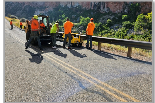
Asphalt Curb Construction Power Plant Road
