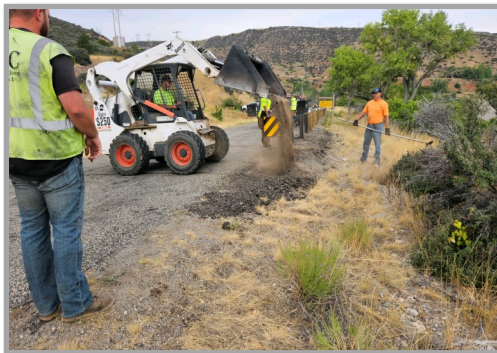
Guardrail Terminal End Pads Power Plant Road
