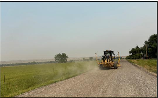
The contractor performs fine grading of the roadway, which is crucial for enhancing the quality of the final paving. Meticulous grading will contribute significantly to the road's long-term performance and durability.
