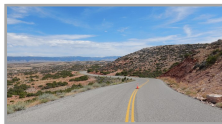
Pavement Markings Devil's Canyon Overlook Road
