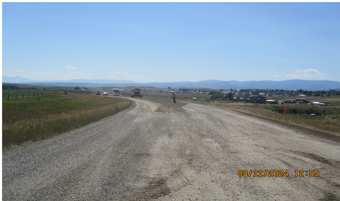
Placing base aggregate near Flathead Creek Br.
