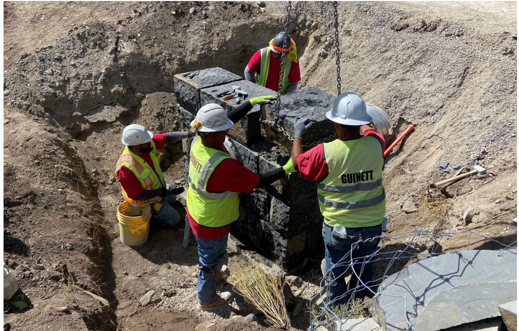
Instillation of Headwalls
