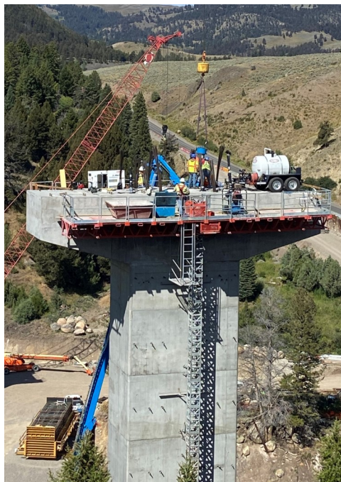
Post Tensioning Pier 3
