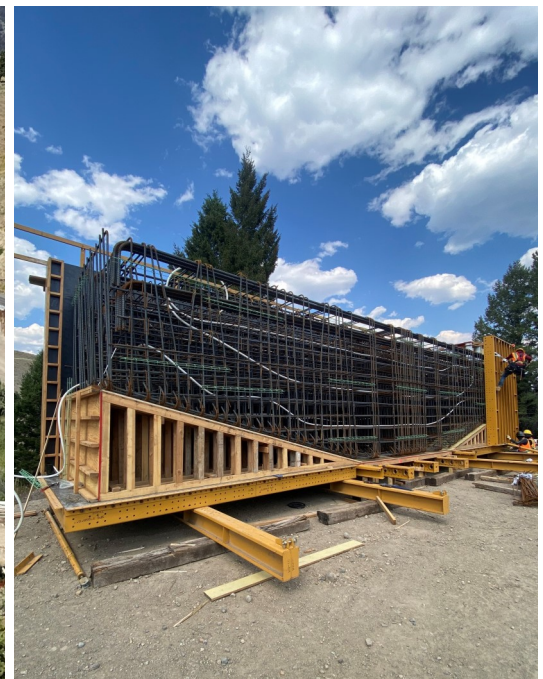
Pier 1 Cap Formwork
