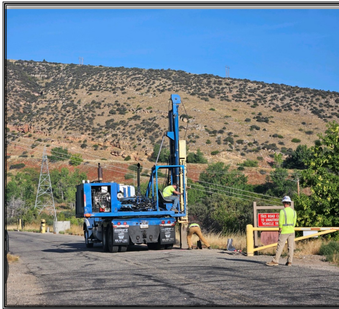
Starting Guardrail Installation on Power Plant Road
