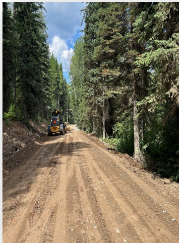
Subgrade Operations on North Fork Road
