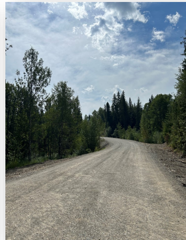
Surface Aggregate Placement on North Fork Road
