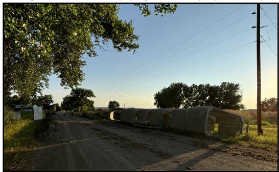
Precast concrete box culverts are staged and ready for installation at the construction site, marking a key milestone in the project's progress. These sections will soon be positioned and backfilled to form a crucial part of the new drainage system.
