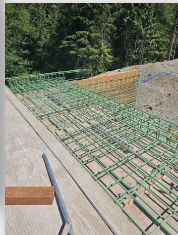
Rebar from top of bridge
