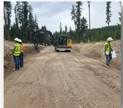
Bottom Photo: Surface Aggregate Course on North Fork Road.
