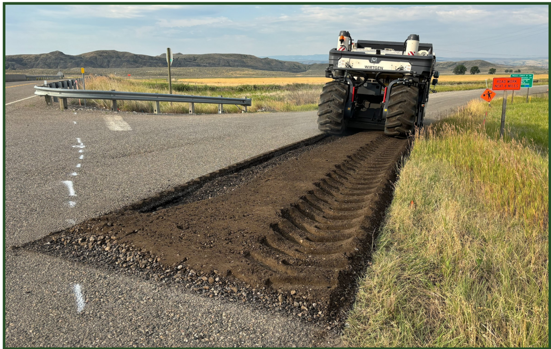
Above, the contractor begins pavement pulverization on Warman Loop Road. The pictured machine performs cold recycling for asphalt as well as soil stabilization.
