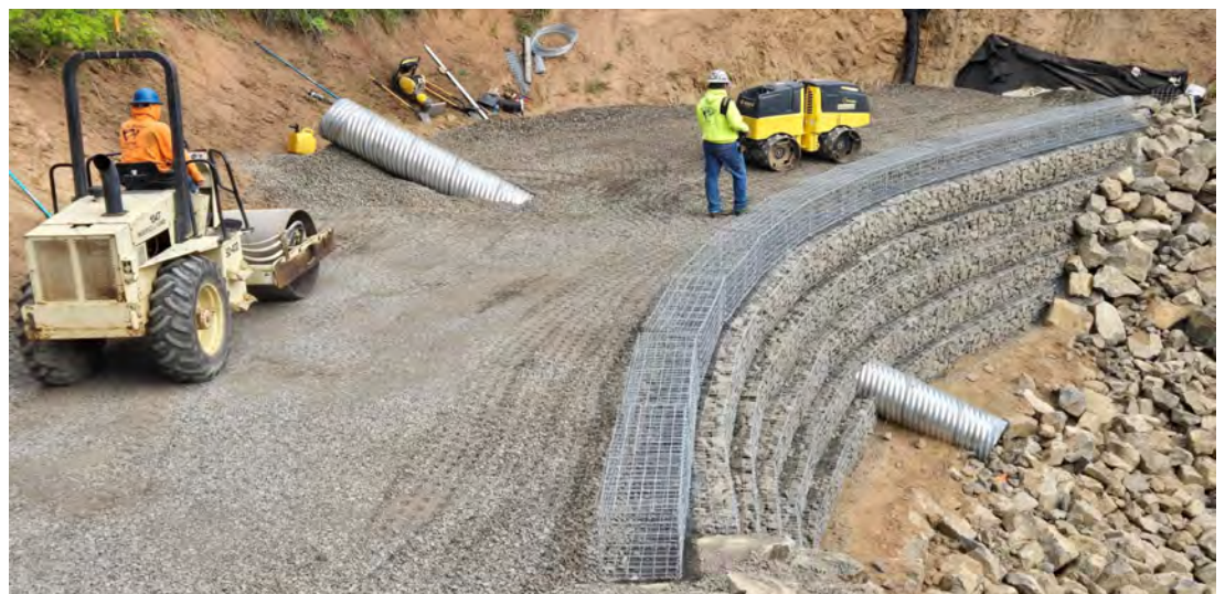
Reinforced soil slope Gabion Faced wall construction FSR5503
