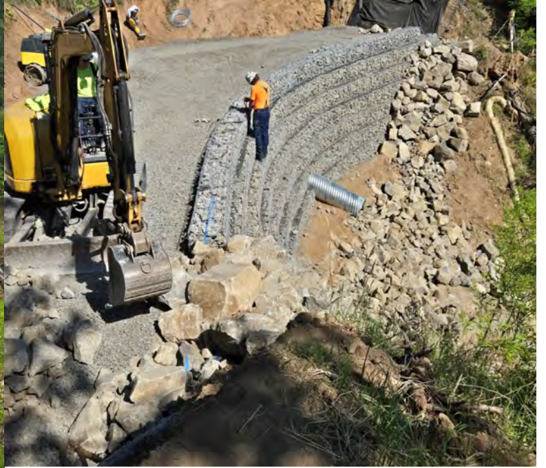
Wall Construction, FSR5503 M.P. 1.28
