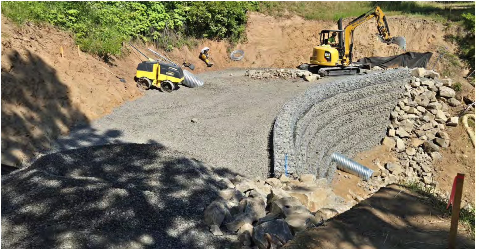
Wall construction, FSR 5503 M.P. 1.28
