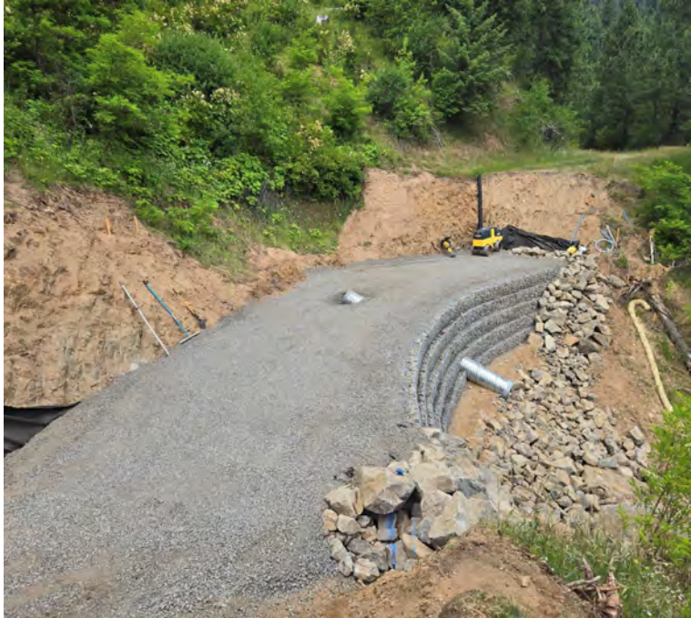
Wall Construction, FSR5503 M.P. 1.28
