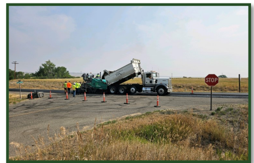
Paving Operations—Afterbay Road
