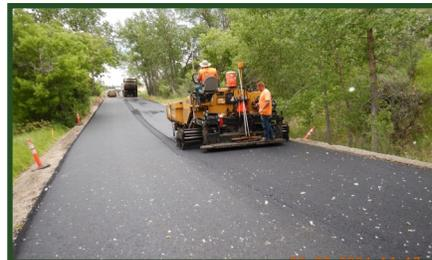
**Type 1A Asphalt Pavement
