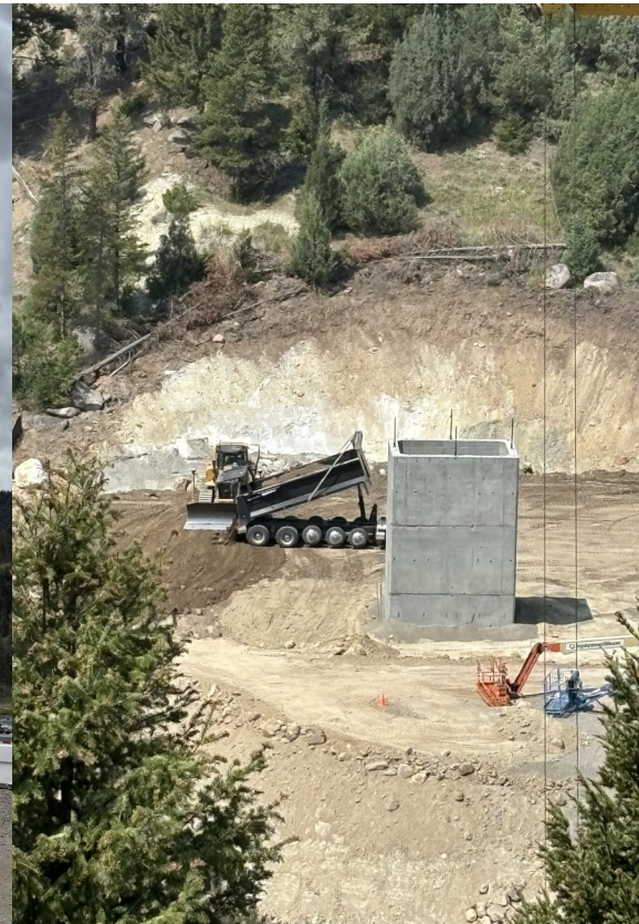
Backfill process at Pier 2.
