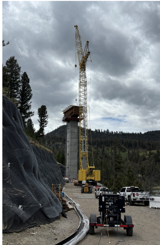
Hanging of the Pier 3 Post-tensioning Strands.
