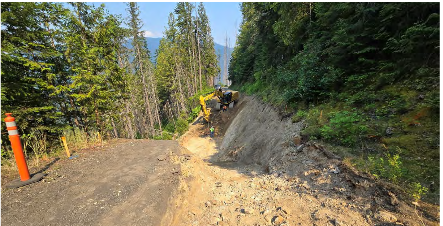
Roadway Excavation, FSR470 M.P. 2.34
