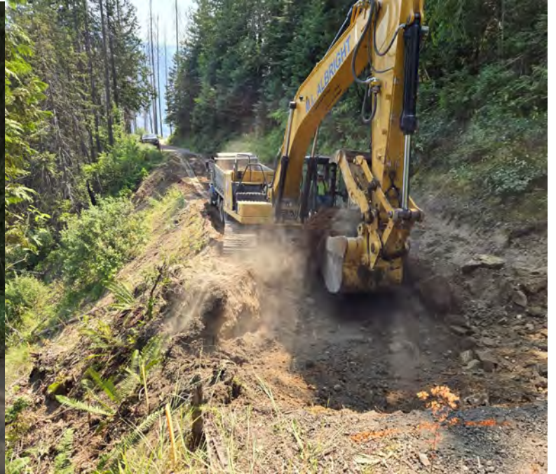
Roadway Excavation, FSR470 M.P. 2.34
