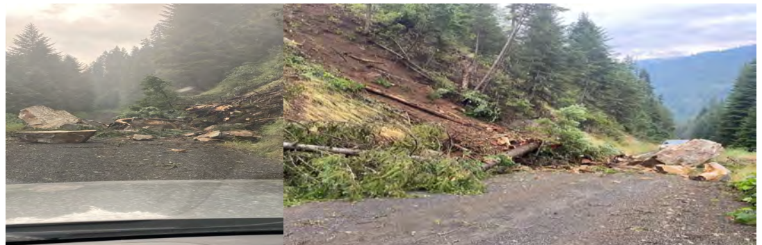
Landslide at M.P. 0.4 FSR469
