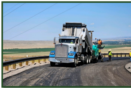
Paving Operations on NPS 313
