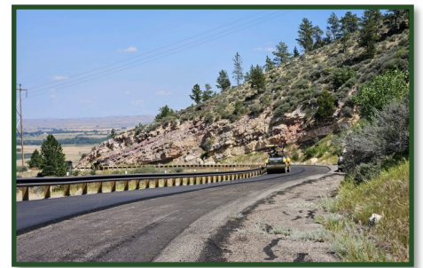
Paving Operations on NPS 313
