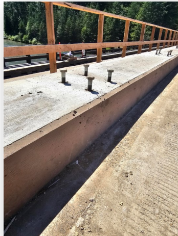
Curb on Bridge
