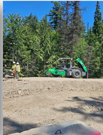
Excavation and Embankment Work
