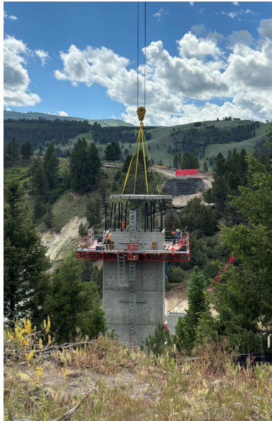
Placement of the Pier 3 stay in place form.
