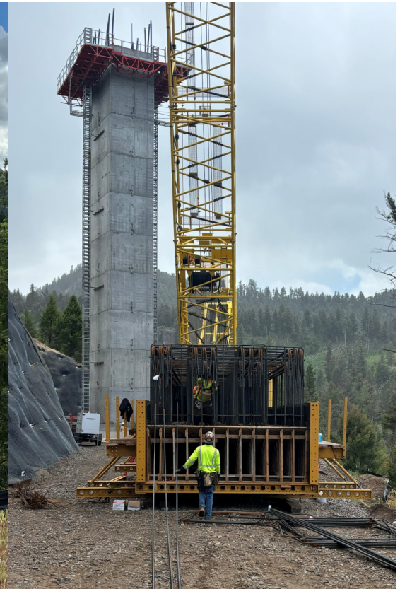
Placement of Rebar within the Pier 3 Pier Cap.
