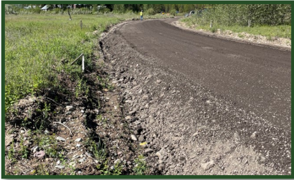
Recycled Aggregate Base placed on Glacier Drive.
