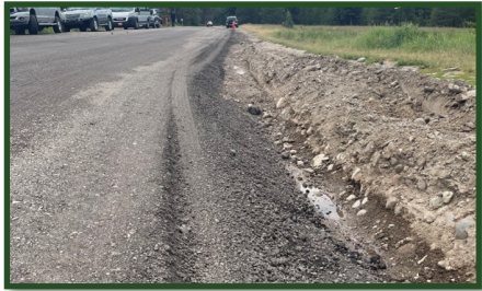
Recycled Aggregate Base placed on Glacier Drive.
