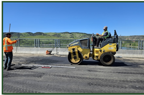
Compacting Type 1(A) Asphalt Pavement patch on Afterbay Road.
