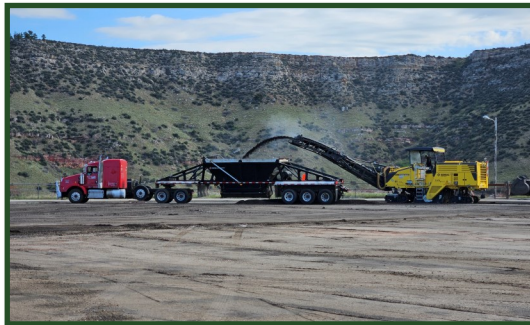
Milling Operations at Upper Ok-A-Beh Parking Lot.
