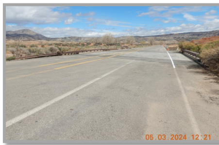
Right Photo – Completed Type 1(B) Asphalt Patch with temporary pavement markings on Bad Pass Road,MP 0.80.
