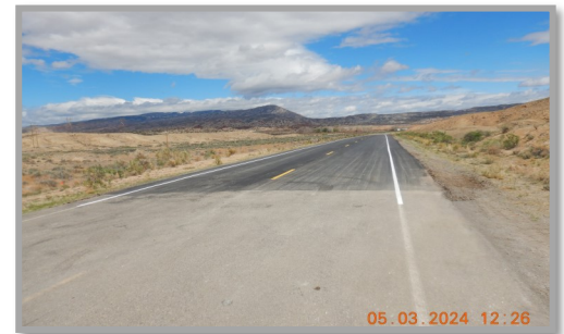
Right Photo – Completed Type 1(B) Asphalt Patch with temporary pavement markings on Bad Pass Road,MP 0.80.
