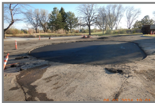
Right Photo- Top Lift Paving on Type 1A Patch at Bad Pass Road, MP 0.80
