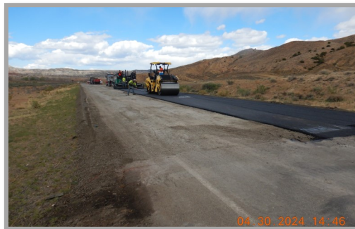
Right Photo- Top Lift Paving on Type 1A Patch at Bad Pass Road, MP 0.80
