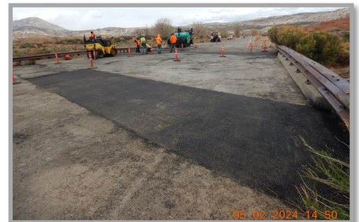
Left Photo: Bottom Lift Paving Type 1A Patch at Lovell Visitors Center Parking
