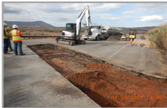
Asphalt Patch Excavation on Bad Pass Road MP 0.08
