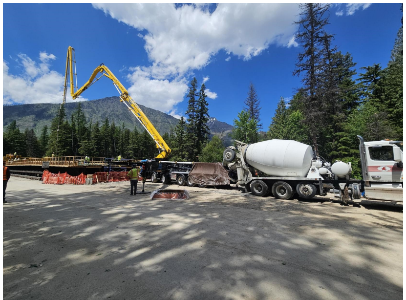
Concrete Mixer and Pump Crane 2nd Pour
