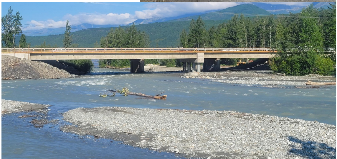
Below: New bridge viewed from the north.
