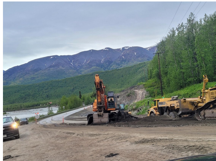
Above: Pavement removal.
