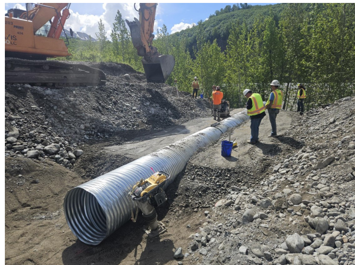
Below: Culvert installation and backfill.
